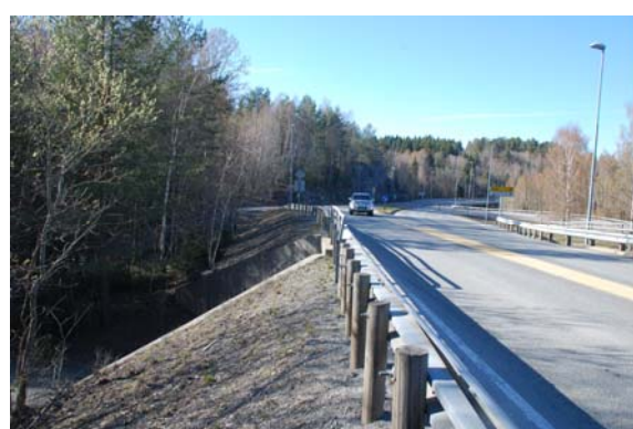
Figur 3-24 Kulvert under fv. 353
